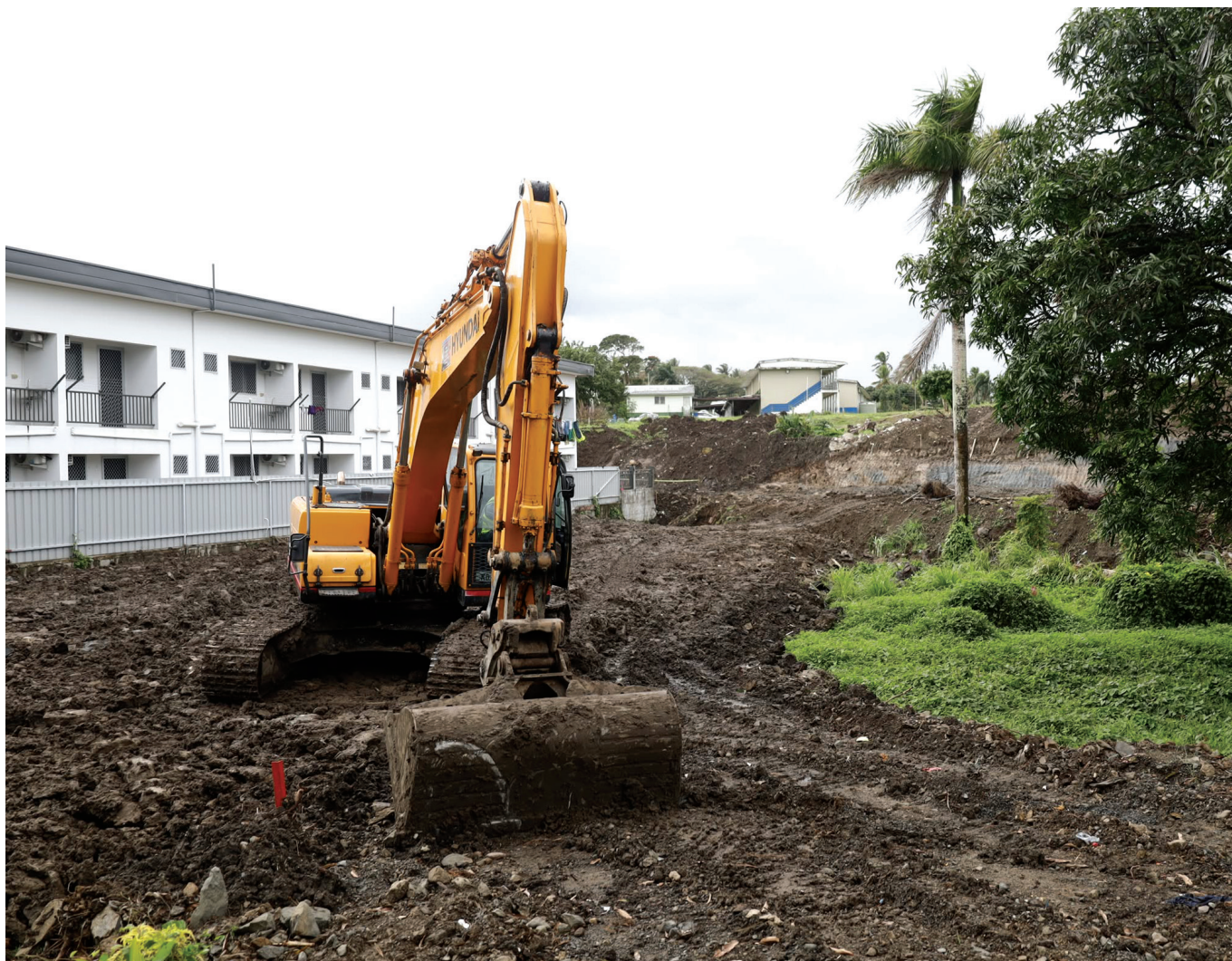
Road construction in Suva
